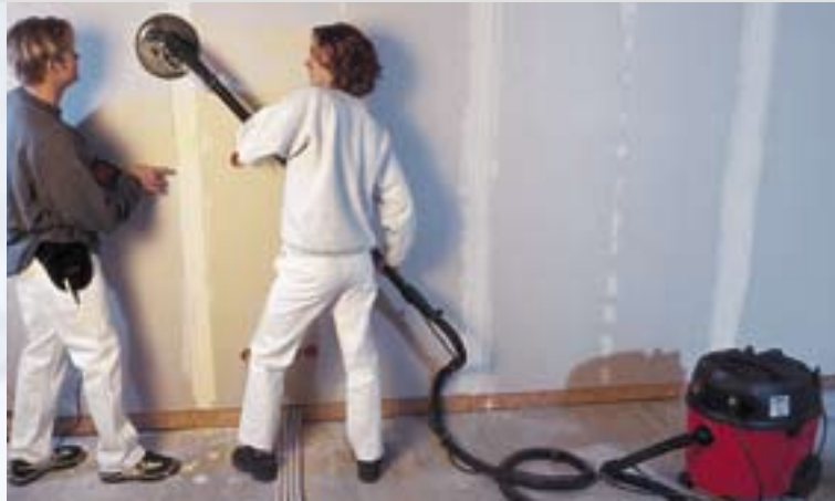
A STRONG TEAM FOR DRY WALL Orbital sander MS 713, long-neck sander WS 702 VEA, industrial vacuum cleaner S 36 and the perforated original FLEX Giraffe sandpapers – all this makes working much easier, quicker, neater, and healthier.
